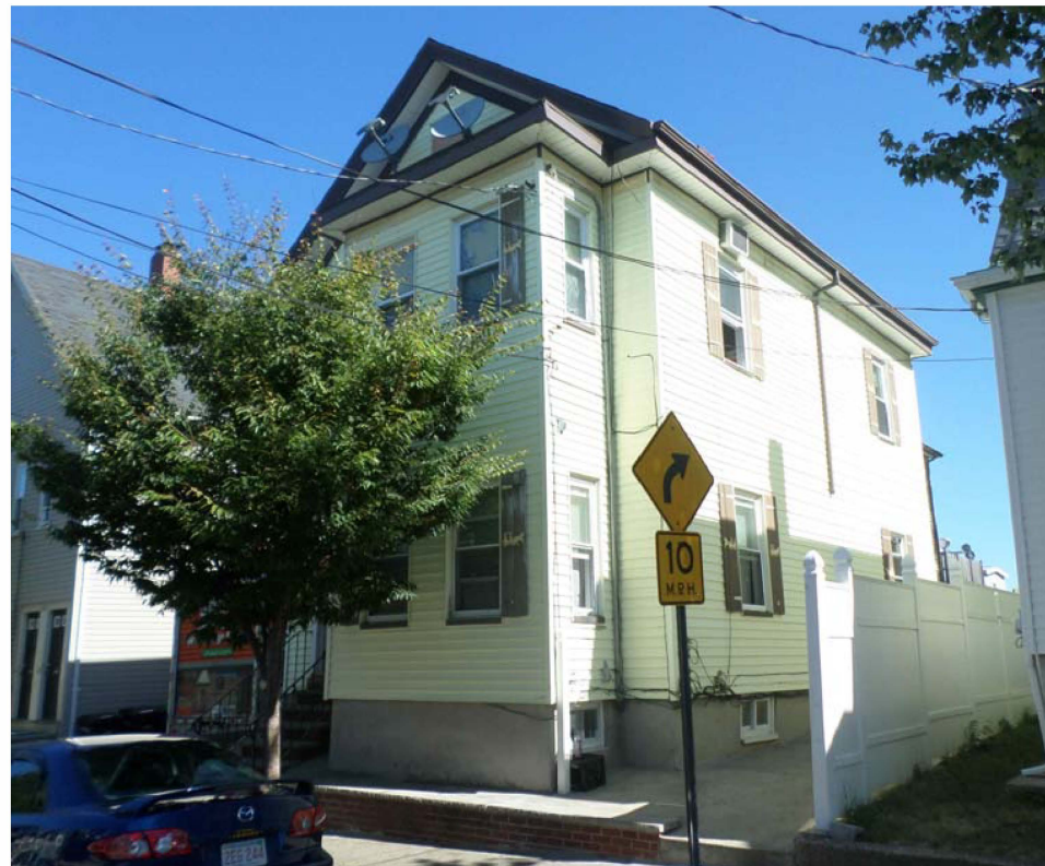
34 SARGENT AVE STREET VIEW FROM SOUTHWEST
